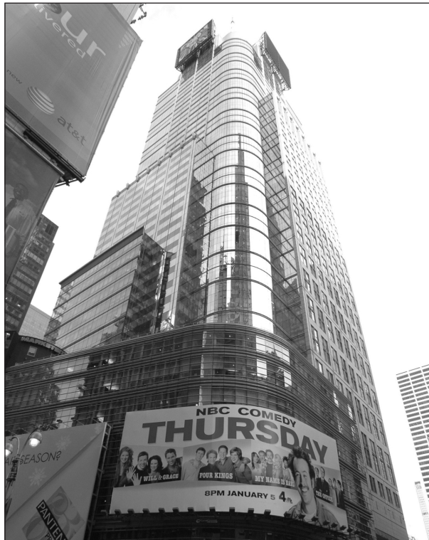
Four Times Square, one of the completed green buildings in New York City.
